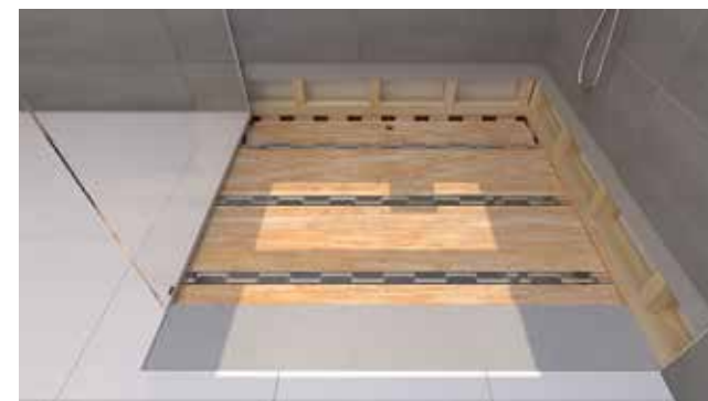
3. Recess Recess the subfloor.
