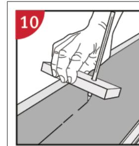
10 Last row (and perhaps also first row): Always keep a minimum width of 2". Place a spacer to the wall before measuring. Mark the plank along the wall. Cut the planks lengthwise including the flexible tongues and install.
